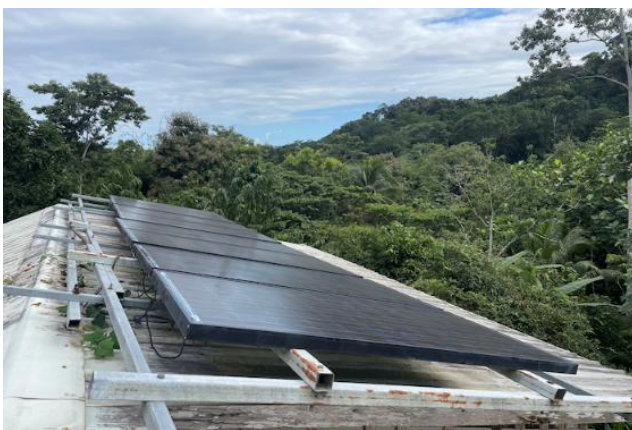
Solar panels mounted on the roof of the third floor of the Main Building
